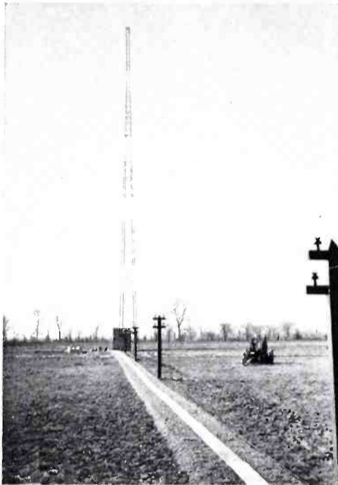
The reflector tower at WBNS
