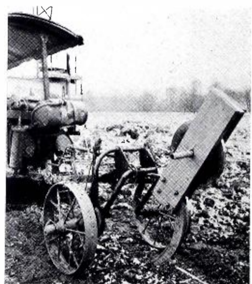
Fig. 2. Laying the ground system for the 400 foot vertical radiator.
