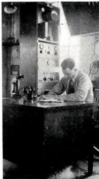
A corner of the control room.
