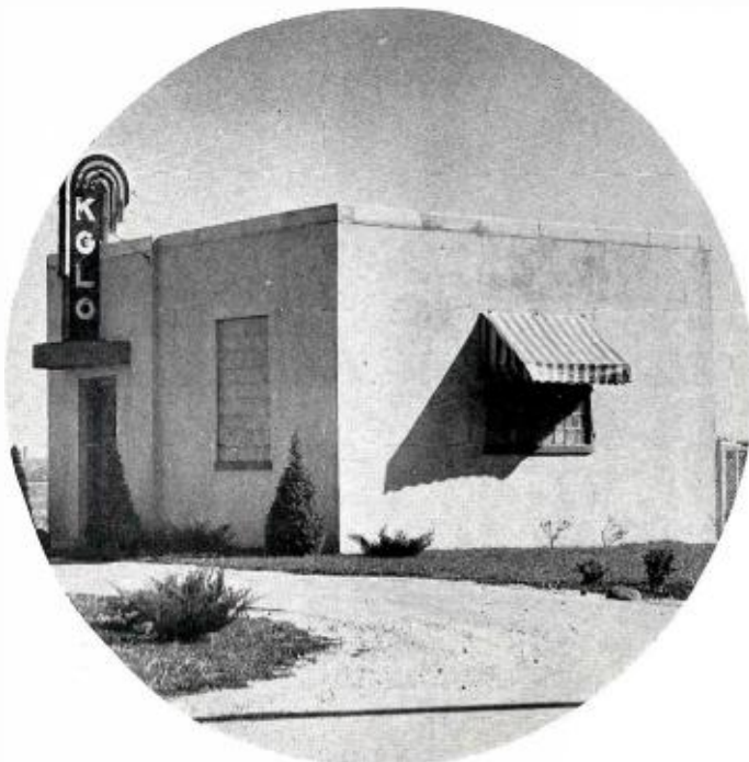
The compact transmitter house.
