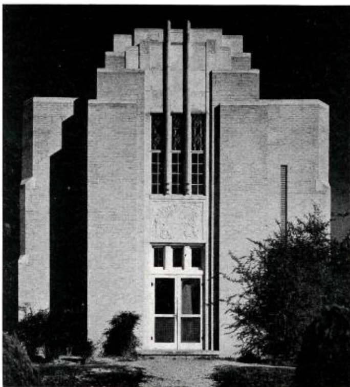
WJDX Transmitter Building. Modern structure houses modern equipment.
