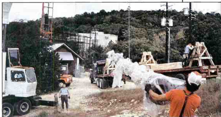
RCA TFU-28DAS high power peanut pattern pylon antenna arrives for installation . . . and is soon mounted atop existing 1290' tower providing KBVO with excellent coverage.
