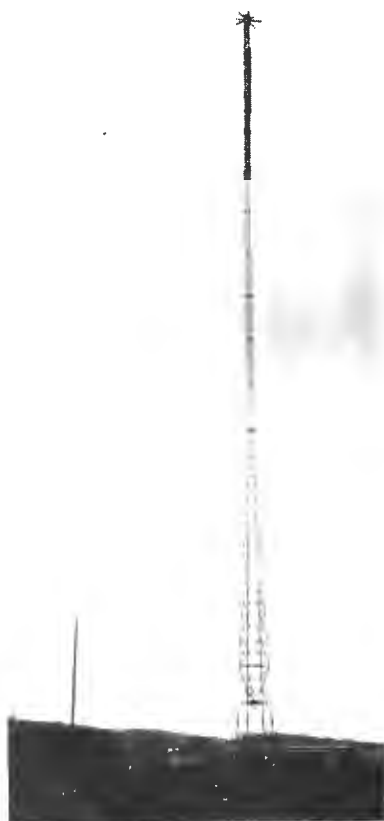
The new half-wave vertical radiator at WDOD
