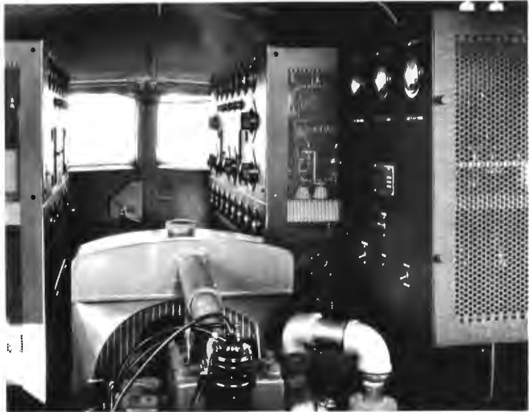
Showing the compact arrangement of equipment in the NBC Mobile Sound Unit.
