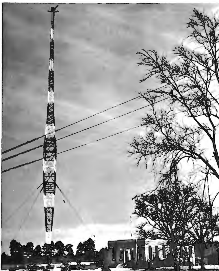
The New Vertical Radiator installed at Station WBT , Charlotte, N. C. This tower is 435 feet high
