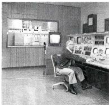
Through the picture window, production control operator has a clear view of transmitter control/metering panels.
