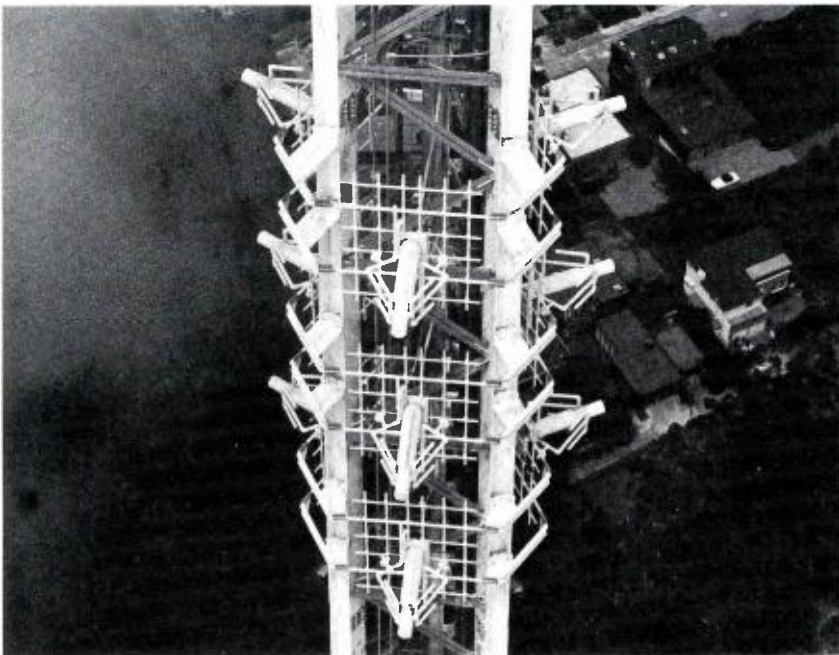
Fig. 13. FM panel, KRON-FM. Mounted on Sutro Tower leg.
