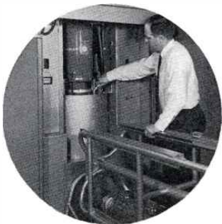
FIG. 8. Disconnect water-inlet hose.
