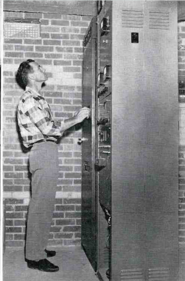
FIG. 3. Chief engineer, Edward Travis, is shown tuning the BTA-250M transmitter. Along side the transmitter is a rack that contains the stations monitors, remote control equipment, and speech input equipment. The transmitter plant is housed in a small brick building 1½ miles south of Brinkley.
