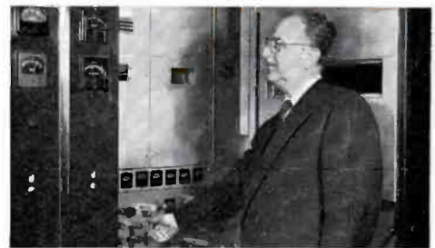
Paul Von Kunits making the only daily adjustment necessary—the carrier level control.
