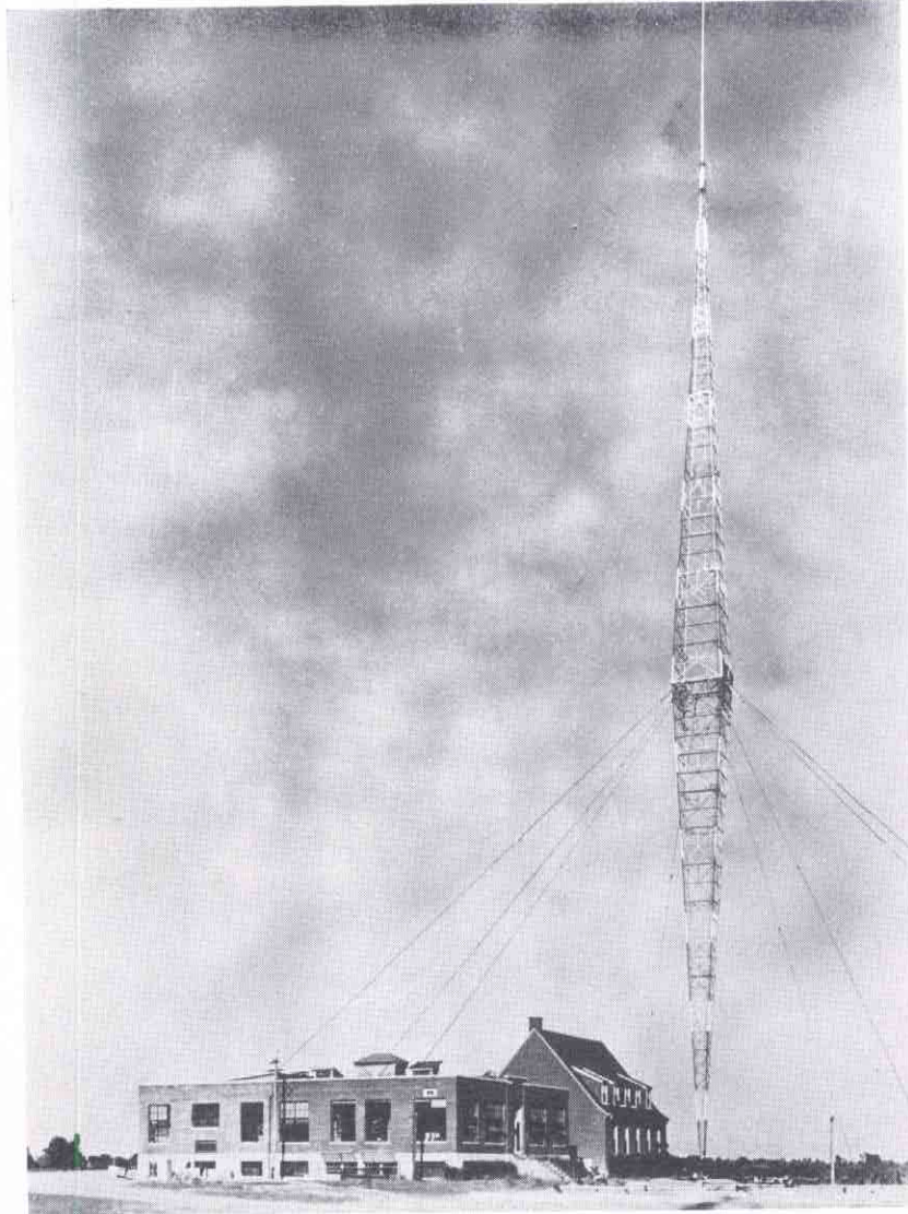
THE NEW 830-FOOT VERTICAL RADIATOR, AND THE STATION BUILDINGS AT WLW
