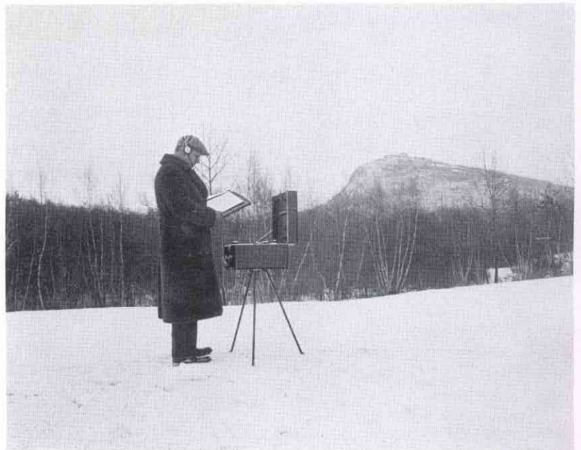
W. L. FOSS, TAKING OBSERVATION ON STATION WBZ WITH RCA VICTOR FIELD INTENSITY METER—MT. TOM IN THE DISTANCE
