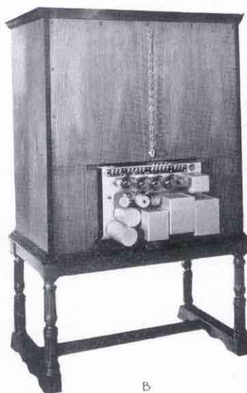
B AMPLIFIER TILTED FOR TUBE INSPECTION
