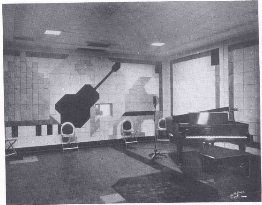
STUDIO B OF STATION WBRE, LOOKING INTO THE "DEAD END." NOTE THE CLEVER MODERNISTIC PATTERN WORKED INTO THE ACOUSTIC WALL TREATMENT. THE WALL SURFACING MATERIAL ITSELF, IN DIFFERENT COLORS AND SHADES, HAS BEEN EMPLOYED TO FORM THESE MOSAIC PATTERNS
