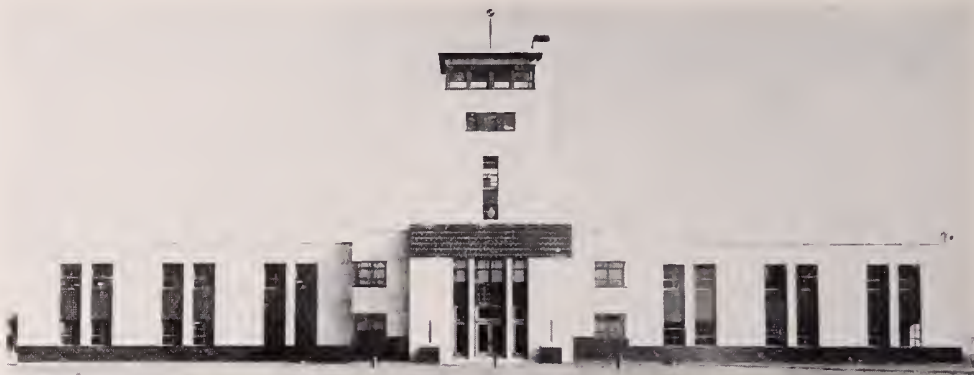
POWERFUL "VOICES"—The attractive new transmitter building near Cincinnati, housing Short Wave Stations WLWR, WLWS and WLWL, believed to be world's most powerful.
