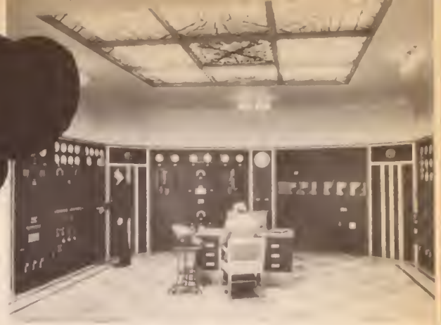
• INTERIOR, WJZ Transmitter, 1936.
